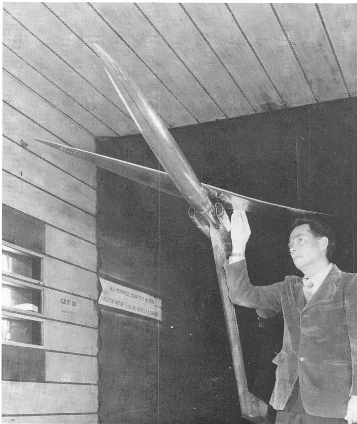
R. T. Jones, shown here with a wind tunnel test model, was the Ames scientist who conceived of the concept of using swept back wings to delay the effects of high speed flight. The design of nearly all modern jet aircraft are based on this knowledge. Photo courtesy NASA-Ames.
